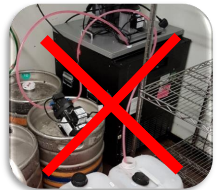
Figure 5 - Remotes side vents blocked by kegs
