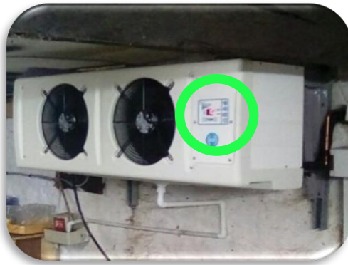
Figure 4 - Cellar Cooling System
